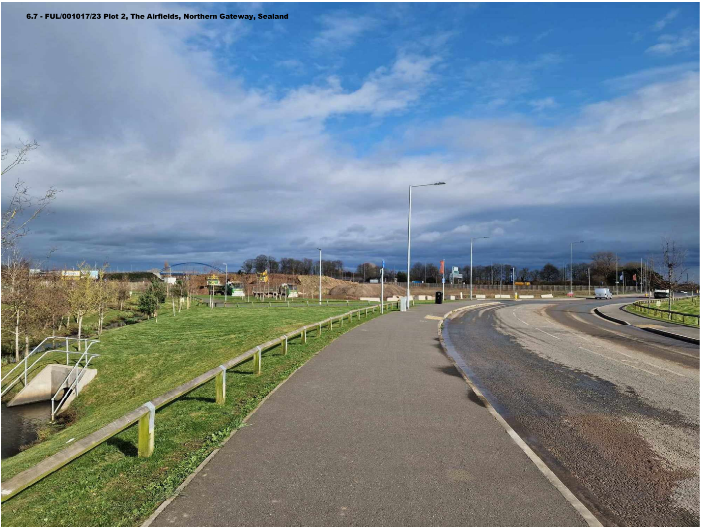
6.7 - FUL/001017/23 Plot 2, The Airfields, Northern Gateway, Sealand
